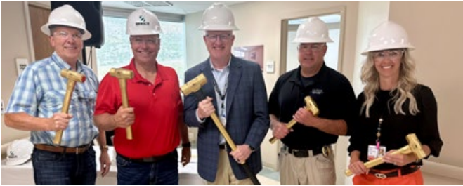
Hospital and community leadership celebrated the start of construction on NNRH's inpatient behavioral health unit in June 2024.
